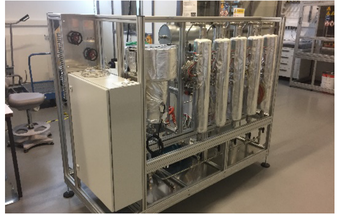
Multi-stage automated gas permeation plant, built by Fraunhofer IKTS.
